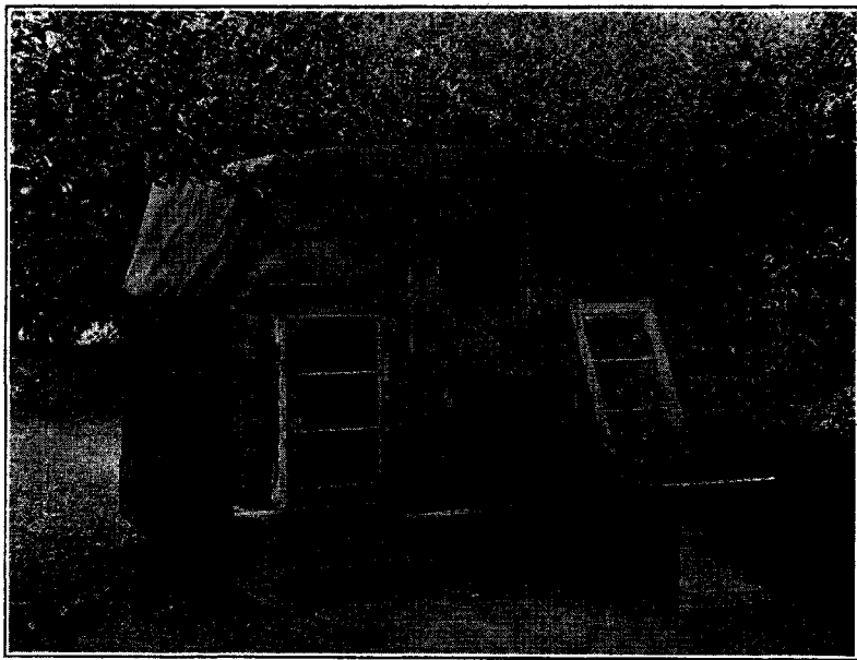
FIG. 12. House made of two piano boxes covered with roofing paper.
