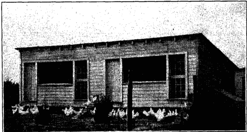
FIG. 5. Shed-roof chicken house having good light and ventilation.
